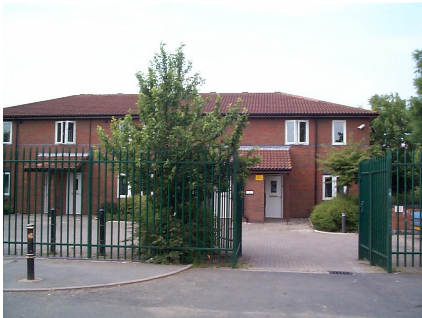
Figure 1. Semi-independent living accommodation
